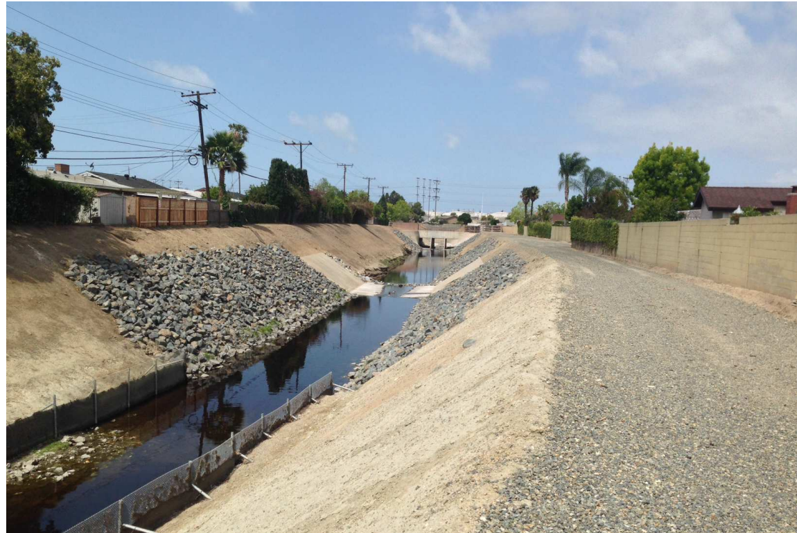
Photograph 5: Looking downstream within the central segment of the channel. California Street bridge is visible in background. Channel is earthen lined with banks that transition between earthen and rip rap. Silt fence repair is shown in foreground.
