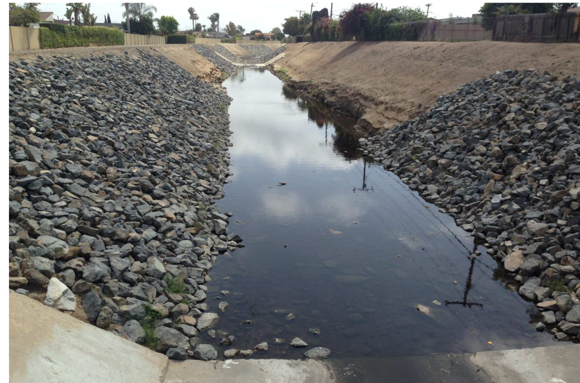
Photograph 4: Looking upstream from the California Street bridge crossing. Concrete transition structure is shown in foreground. Channel supports an earthen bottom with banks that transition between earthen (undercut) and rip rap-lined.
