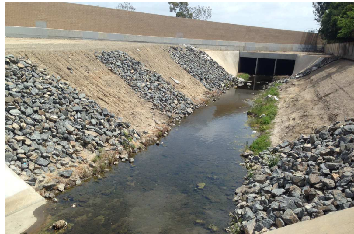
Photograph 8: Looking at the upstream-most segment of the channel from the New Hampshire Drive bridge crossing. Concrete transition structures are shown in foreground and background. Channel supports an earthen bottom with banks that transition between earthen (undercut) and rip rap-lined, with 2'x100' herbaceous weedy vegetation at toe of slope.
