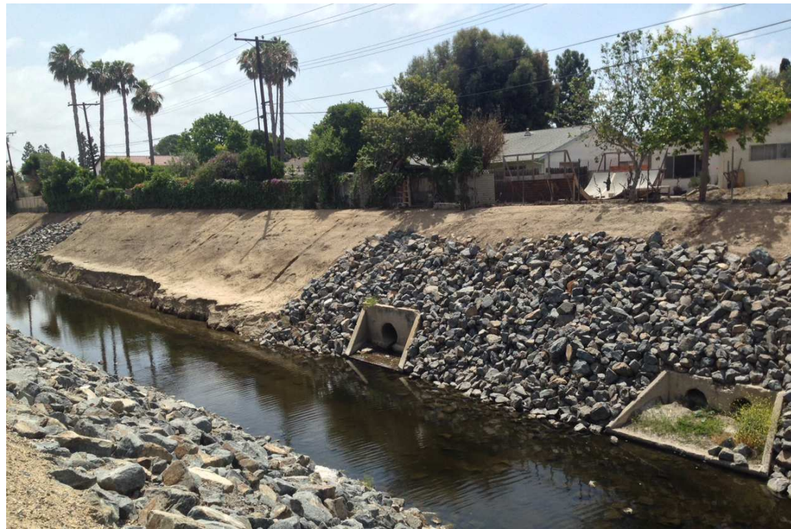
Photograph 7: Looking further upstream within the central segment of the channel. Two outfall structures discharge nuisance flows from surrounding urbanized areas into the channel. Channel is earthen lined with banks that transition between earthen and rip rap.
