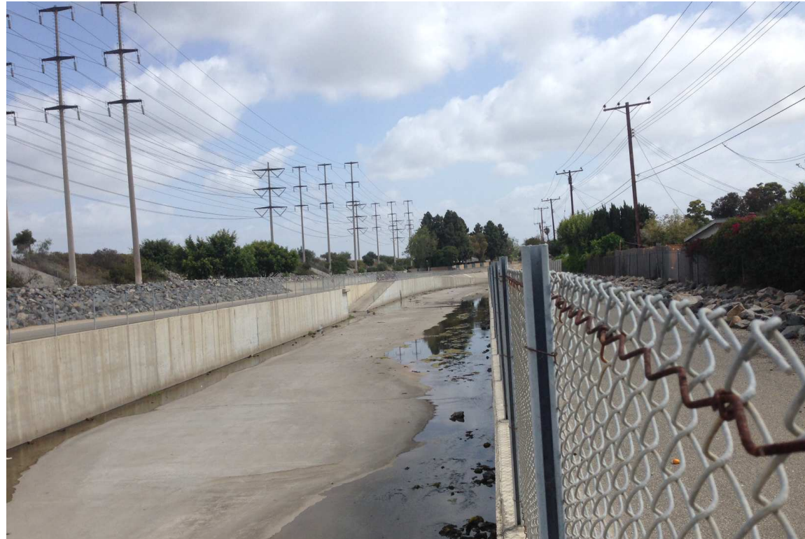
Photograph 1: Looking upstream at the downstream-most segment where the channel is confined entirely within a concrete bottom and concrete vertical walls.
