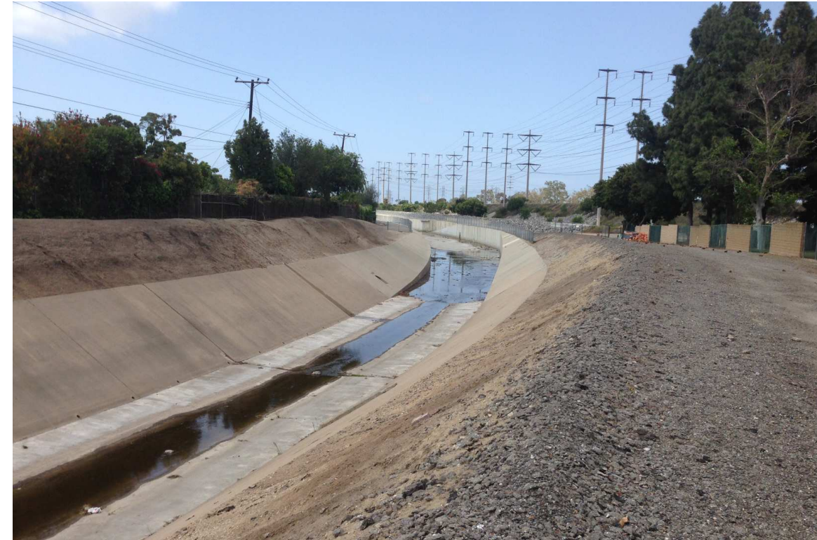
Photograph 2: Looking downstream at the point in the channel as it turns south to parallel the Santa Ana River. The channel bottom and lower section of the banks are concrete lined. Maintenance access road is shown to the right.
