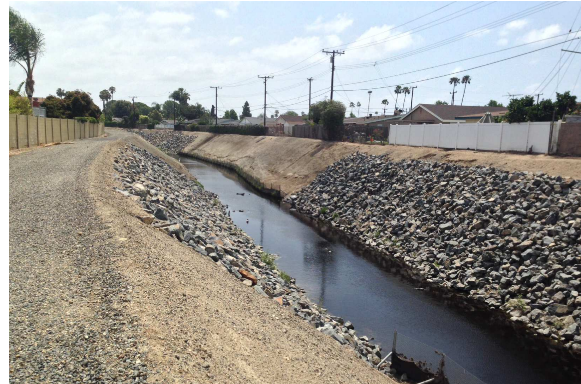
Photograph 6: Looking upstream within the central segment of the channel. Channel is earthen lined with banks that transition between earthen and rip rap.
